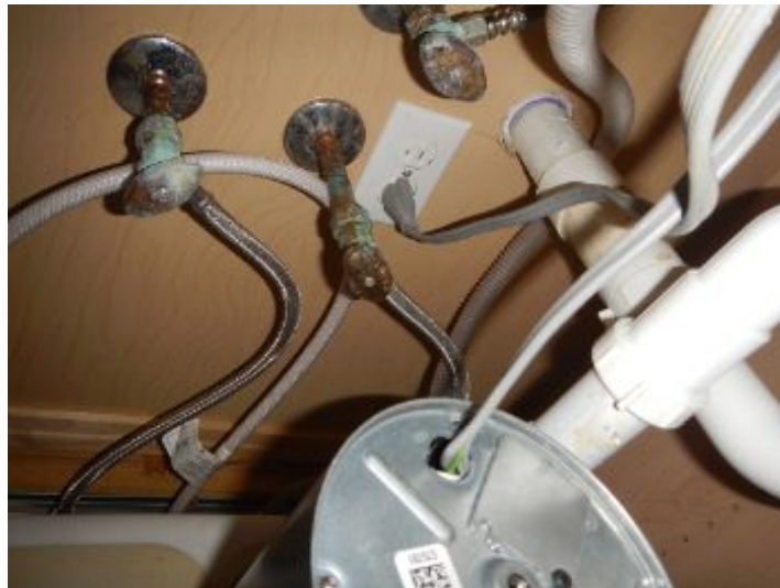
Unit was locked up at time of inspection
