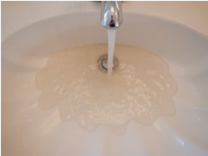
Rust colored water should be evaluated by a licensed plumber
