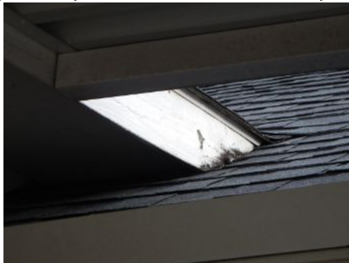
Wood rot on fascia over back porch
