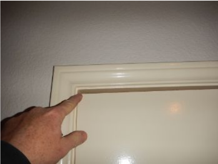
Back door is out of align
